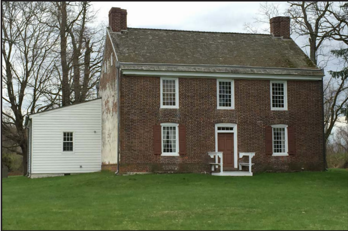
Photograph 1.3. The Brearley House in April 2016. View facing south showing the front of the 1761 house. The probable late 17th – early 18th century basement/cellar hole lies immediately in front of the left half of the façade. (Photographer: Ian Burrow).
