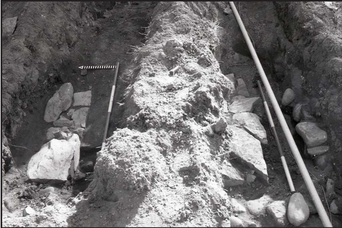
Photograph 3.13. Trenches A, B. View showing possible fireplace foundation exposed in contractors' excavations, about 12 feet west of the 1761 house. (Photographer: Vivian Braubitz, April, 1999) [Hunter Research Inc. Neg. 98053/21:22]
