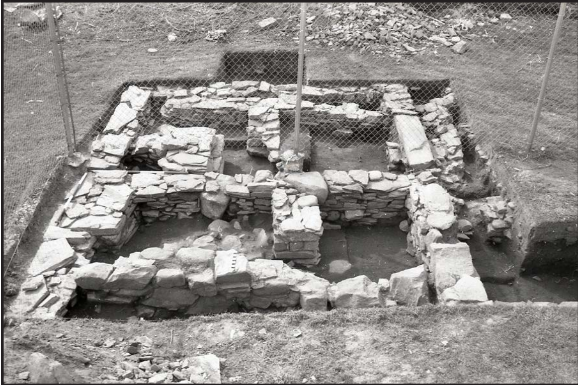
Photograph 3.6. The north and south kitchen wing sections as fully excavated, but prior to the exposure of the northern portion of the north wing, which took place after the removal of the security fence (see Photograph 3.1). The late 18th/early 19th century fireplace foundation is in middle view with bake oven remains in left middle view. The 19th century cross wall is at bottom of view. View facing south. (Photographer: Eric Landis, April 1999). [Hunter Research Inc. Neg. 98053/16:7].
