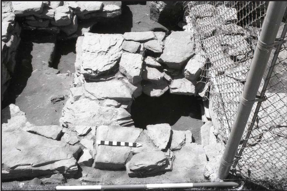
Photograph 3.3. The foundations of the late 18th/early 19th century beehive bake oven. View looking west. This was bonded into the south wall of the north wing (to the right of the fence), and was abutted by the east wall of the south wing addition, visible at bottom left south of the north arrow. (Photographer: Eric Landis, April 1999) [Hunter Research Inc. Neg. 98053/14:14].
