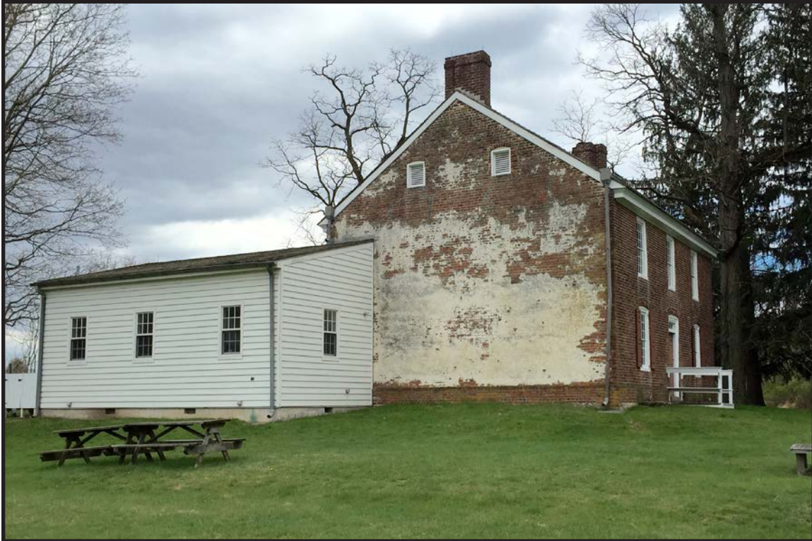
Photograph 1.4. The Brearley House in April 2016. View facing southwest showing the partially stuccoed east wall. The 1761 date is picked out in glazed headers in the gable just below the attic windows. (Photographer: Ian Burrow).
